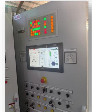
New PLC Based Electrical Control Panels
