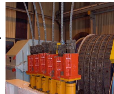
Reliance glands with tensioning jacks
